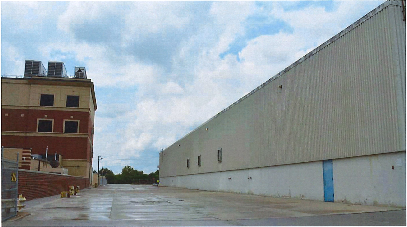
FIGURE 8. FROM KENTUCKY AVENUE, THIS VIEW SHOWS THE APPROXIMATE PATH OF HENRY STREET WITH DIAMOND CHAIN TO THE NORTH (RIGHT) AND INDY TELCOM CENTER TO THE SOUTH (LEFT).
