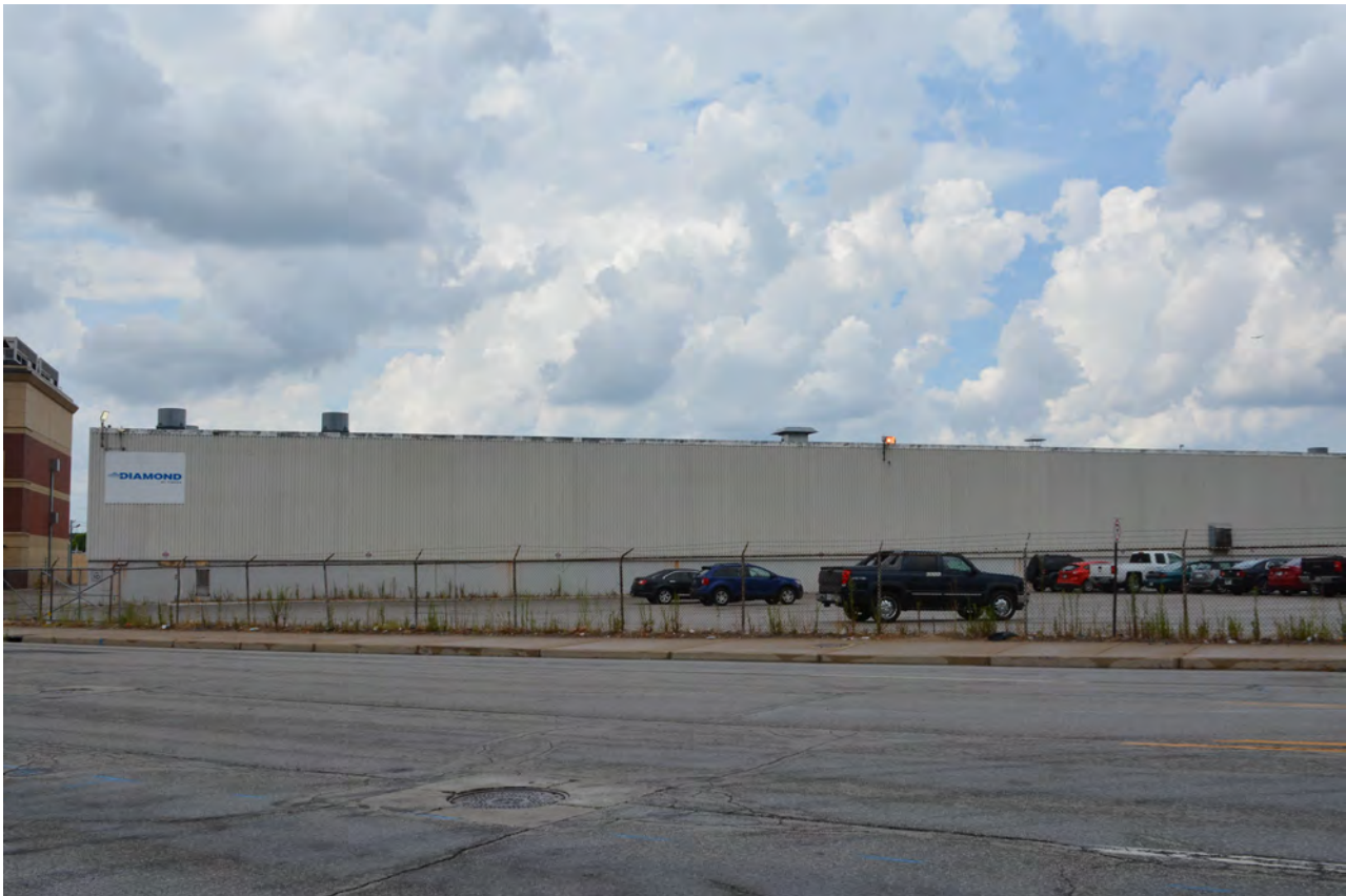
8. This circa 1970s addition is part of the Diamond Chain Company Complex.
