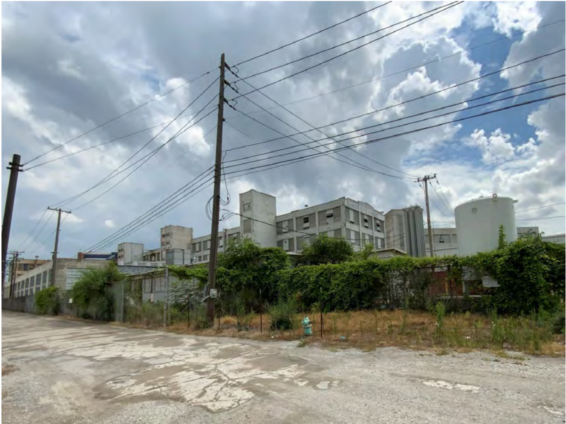
10. Looking southeast on the northside of the Diamond Chain Company Complex (non-façade elevation).
