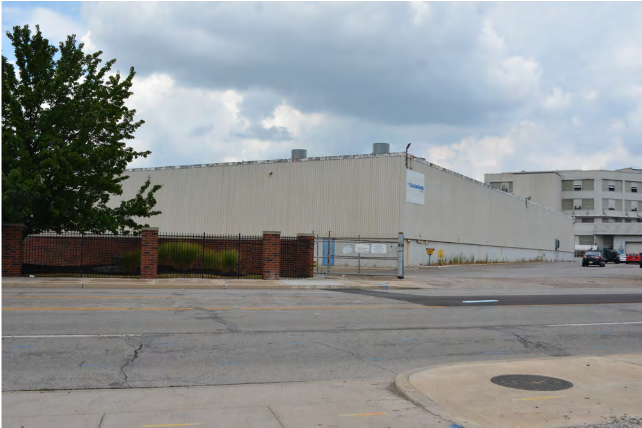
Figure 6. The southern addition was added circa 1970 (looking west-northwest near Henry Street).
