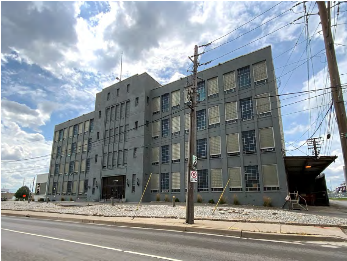
Figure 5. The oldest portion of Diamond Chain dates to 1917 (east elevation).
