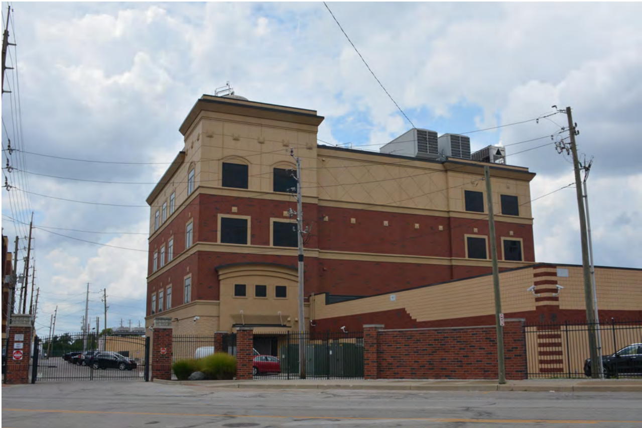
5. Looking northwest across Kentucky Avenue to a non-contributing building (550 Kentucky Avenue, c. 1990) within the APE.
