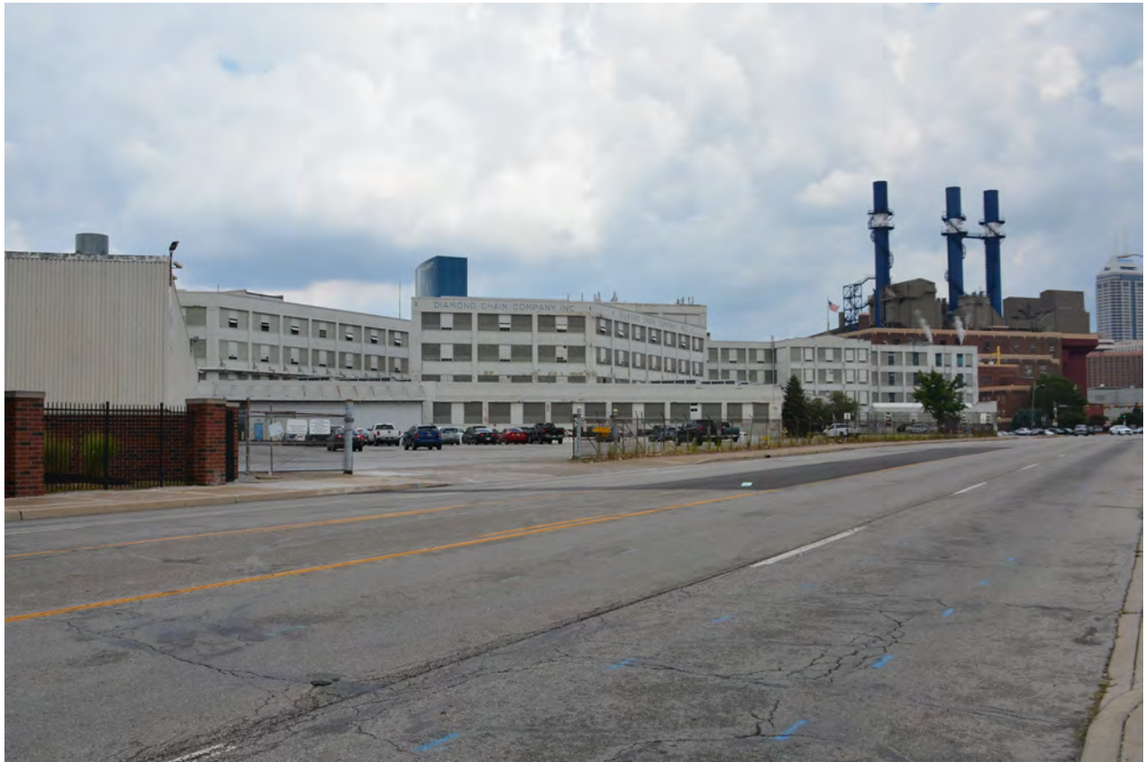
9. Looking northwest along Kentucky Avenue showing the circa 1940s addition to the Diamond Chain Company Complex (Center of photograph).
