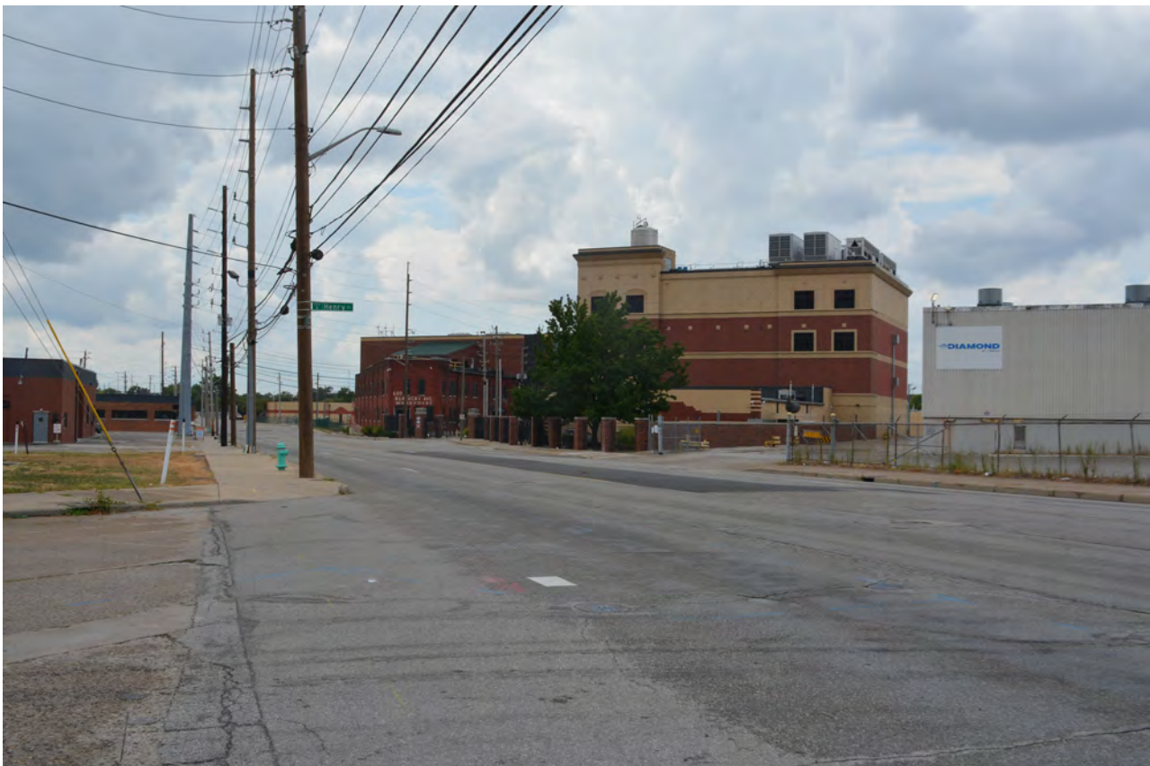
6. Looking southwest along Kentucky Avenue to the proposed project (right side of photograph).
