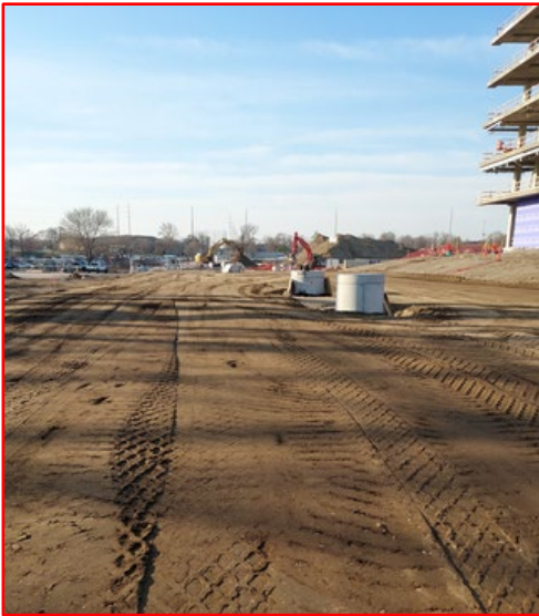
Embankment construction on South White River Parkway
