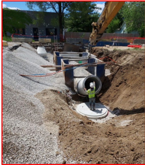
The 42-inch storm sewer along Holly Street
