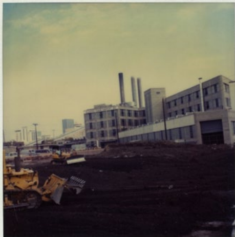
10/16/80 Backfilling and compaction - south side of bldg.
