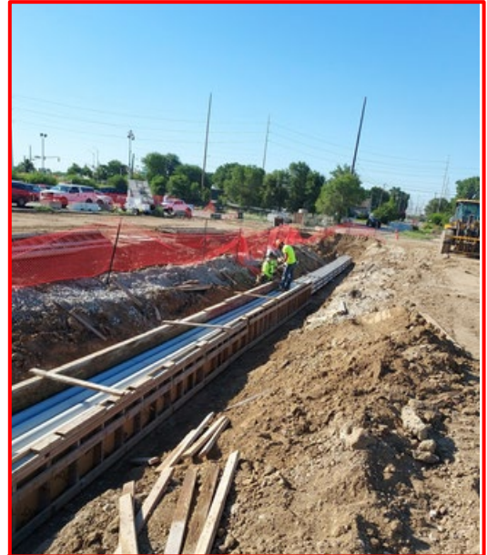
AES Duct Bank, south of Henry St. on SWRP, looking south
