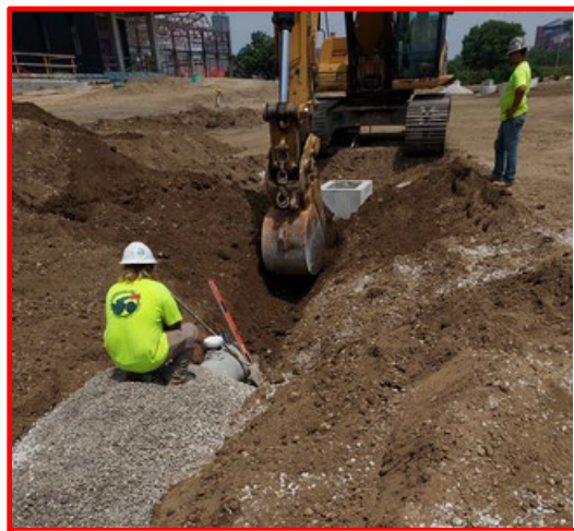
Installed curb inlets on Henry St.
