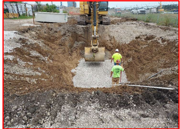
Preparing to install the AES vault near Arbor St.
