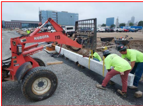
Dry setting the granite curb along Holly St.
