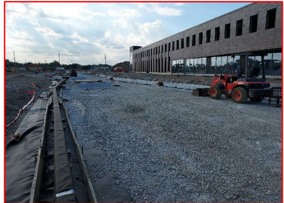
Installing the granite curb along Holly St.
