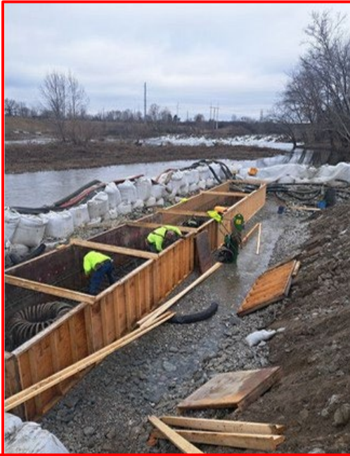
Setting reinforcing steel in Pier 5 footing, looking north
