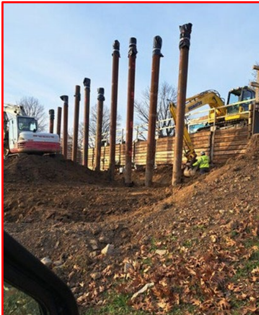
Crews work on End Bent 1 for the Henry Street Bridge.
