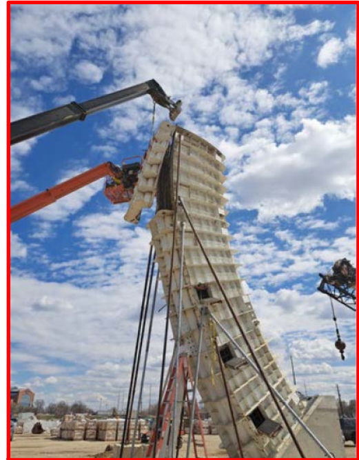
Crews set the formwork for the concrete ring mock-up
