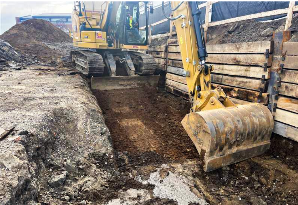
Mechanically stripping overburden fill to uncover shafts
