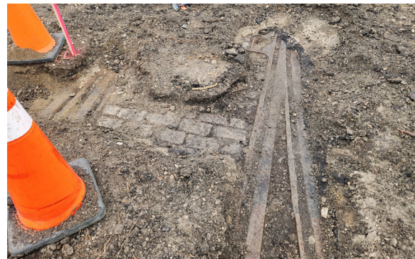
Figure 15. Traction depot rails and pavers uncovered during Project Area site preparation
