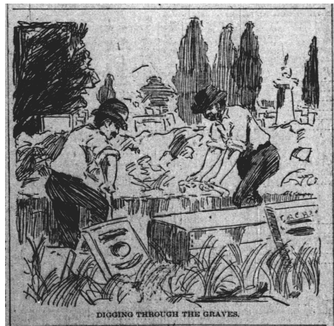
Figure 9. Sketch of burial exhumations during the 1896 sewer installation through Greenlawn Cemetery
