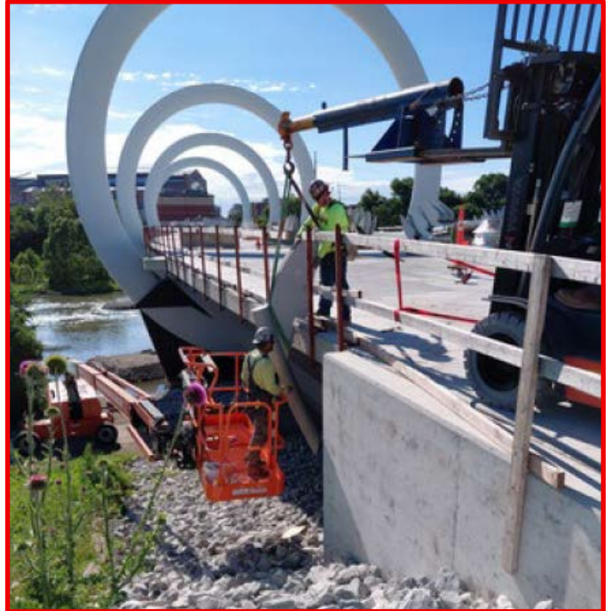
Crews begin installing the pedestrian rail on the north side of the bridge.
