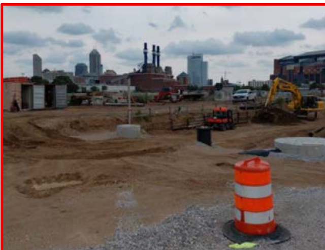
Installing the storm sewers is underway east of the bridge.
